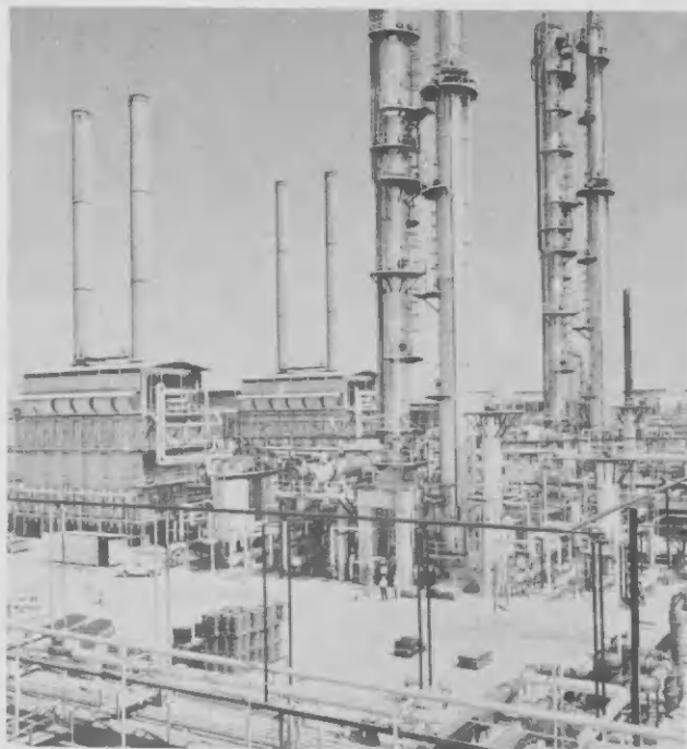
Completed Hydrogen Plants north of Powerhouse No. 1. Plantas Hidrogeno completa, noord di Powerhouse 1.
